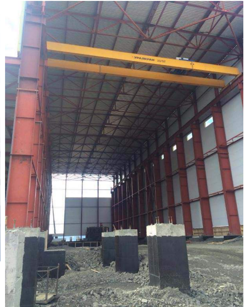
Foundations for tailings discharge conveyor and installation of overhead crane
