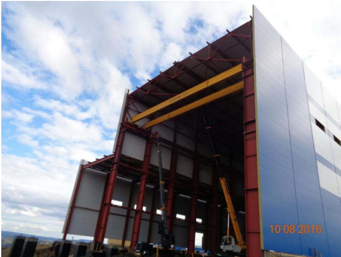
Main Plant, installation of weather shielding
