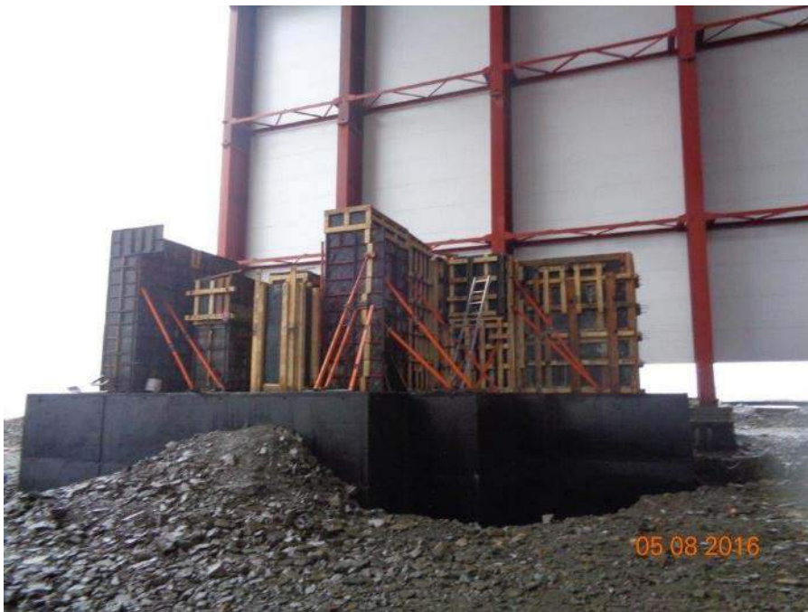
Ball Mill foundation
